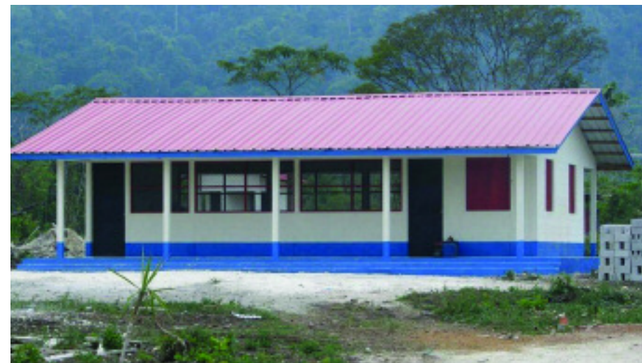
Residents will benefit from a new school in the Santa Rosa Community Resettlement in the Adjacency Zone. Below: Sergio Benítez, Director of the Office of the General Secretariat in the Adjacency Zone, carries out a verification with the help of GPS equipment
