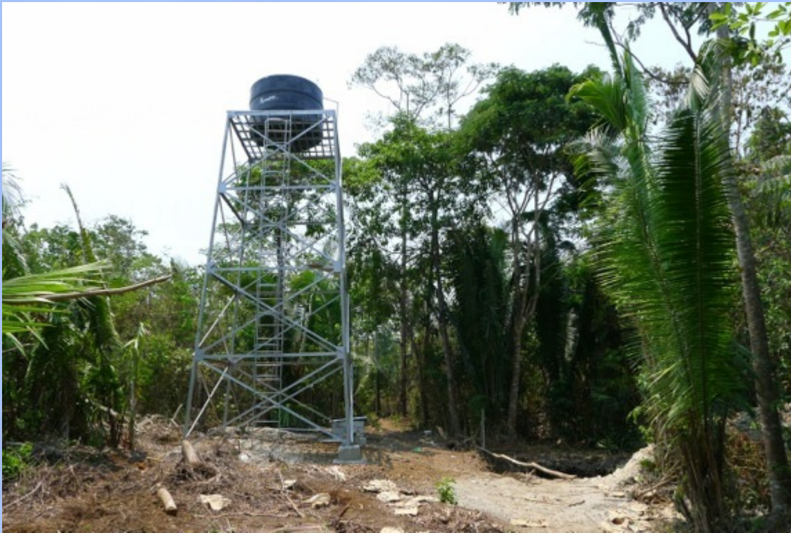
A 5,000 liter reservoir was installed on a tower
