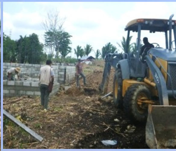
Commencement of Housing Project
