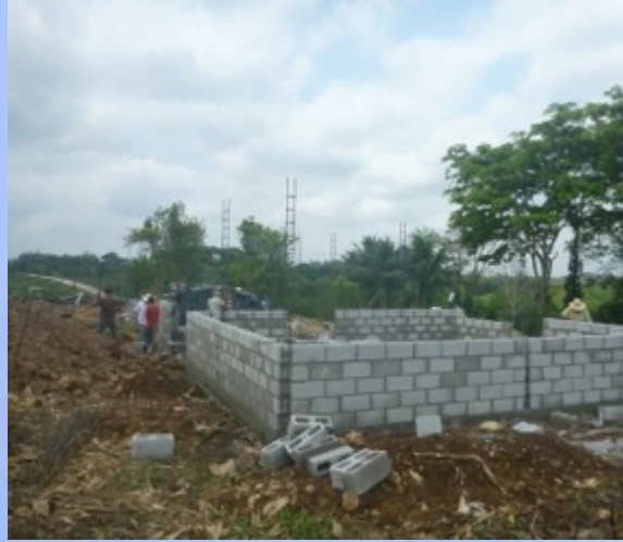
Construction Process – Housing Project
