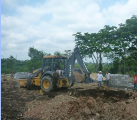
Excavation for septic tanks / water disposal
