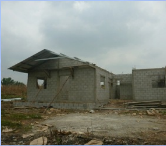
Construction Process – Housing Project
