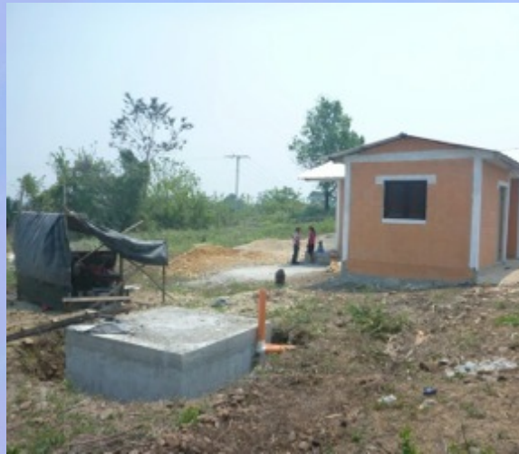
Septic tank project finalized
